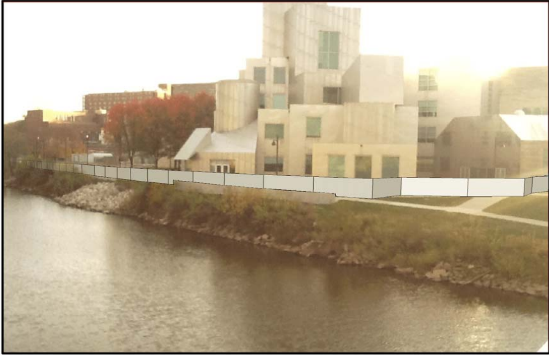
Schematic image of proposed removable flood wall installed at site. Flood condition not shown.
